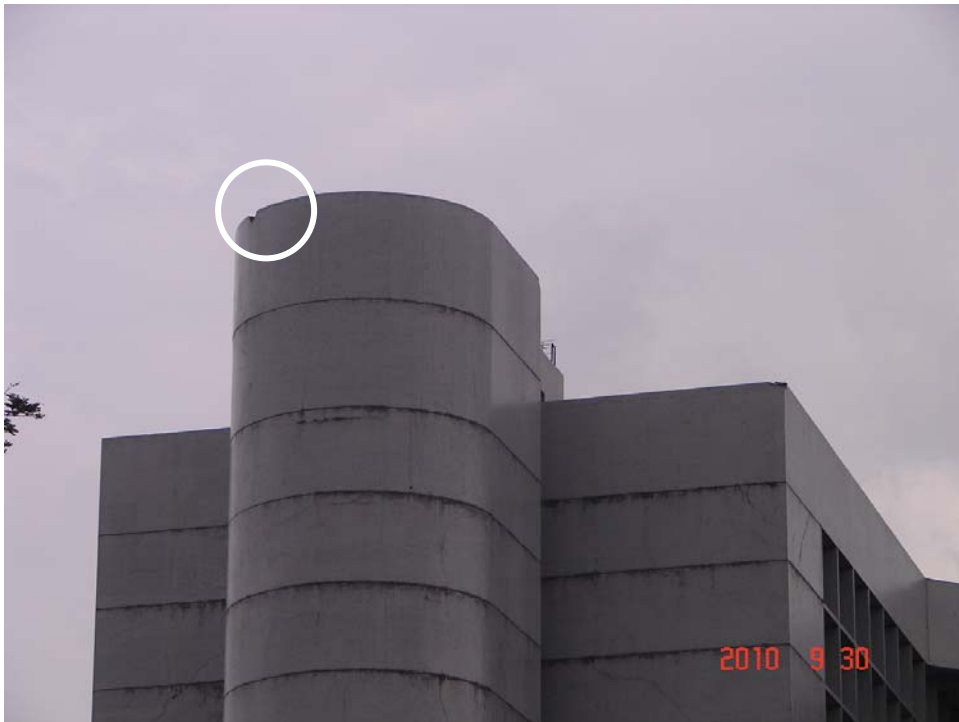
Figure 16: A bypass on the curved edge of the parapet wall on the west wing of the DCS building.
