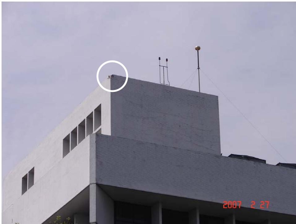
Figure 14: The bypass nearest to the Dynasphere air terminal about 10 metres away.
