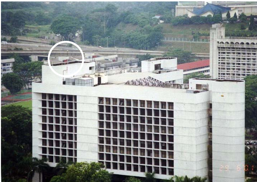
Figure 12: The DCS building photographed from another building which is located to the North-West. The Dynasphere air terminal (circled) was installed at the centre of the building.
