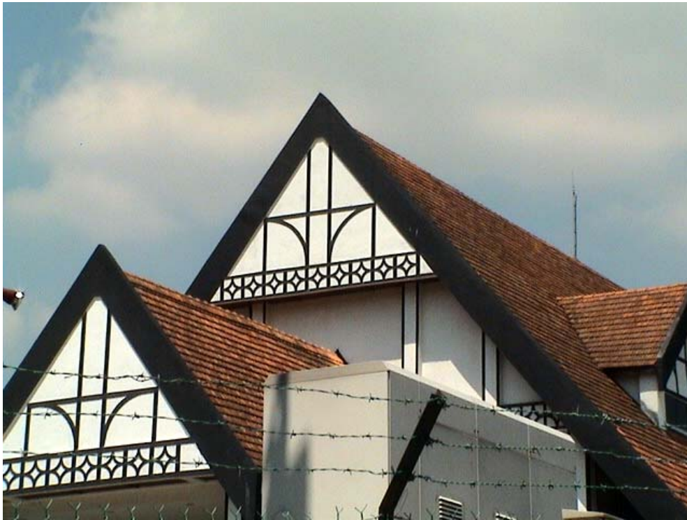
Figure 10: The repaired façade and the new Spanish made ESE air terminal in 2004.
