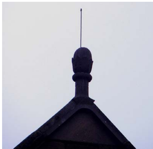
Figure 6: Another view of the correctly positioned Franklin rod on top the roof of the main building.
