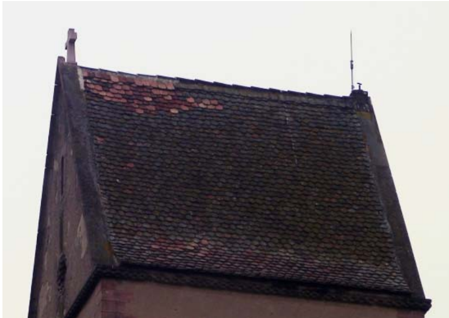
Figure 5: The repaired bell tower of the Saint Pierre and Paul church in Sigolsheim taken a year after the lightning strike incident. Note the new stone cross and the absence of any change in the height of the ESE air terminal.
