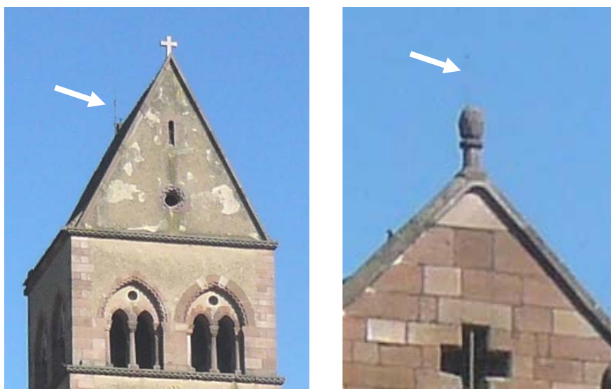
Figure 2: Magnified pictures of the church reveals a Helita Pulsar 25 ESE lightning air terminal (left) and a Franklin air terminal (right) installed on roofs of the bell tower and main hall respectively.
