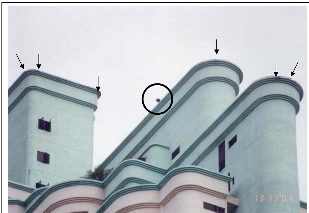
The Villa Putri apartment building in Kuala Lumpur was damaged (arrowed) by lightning at 7 different places on the roof. In spite of this building being a subject in a conference paper in 2000, the sales engineer still informed the building manager in 2002 that the building was free from lightning strike damages. One of the two Australian ESE air terminals can be seen above (circled).
