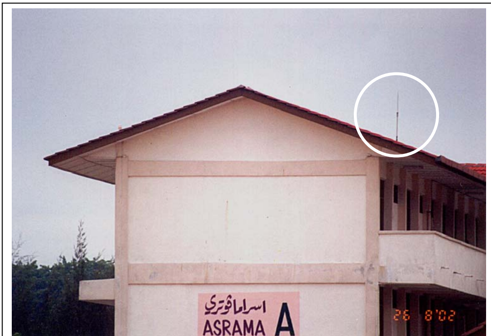
A French-made ESE air terminal (circled) was installed on the roof of the adjacent building (Asrama A) which is about 20m from the lightning strike damage. According to the vendor's product description, this device provides coverage of about 50m radius i.e. to "protect" both blocks A and B. This failure is just another example that the sophisticated lightning protection system does not work.
