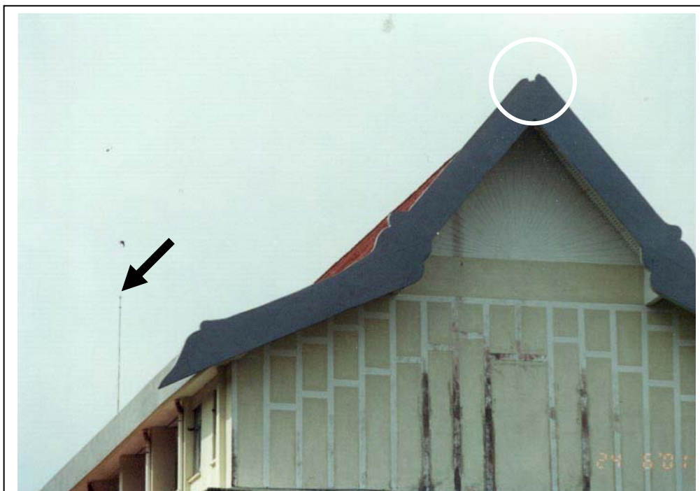
One of the UTM buildings in Skudai that had its façade damaged (circled) by lightning. An undamaged façade would have a sharp pointed apex. Several other similar buildings had been struck also with the damage in varying sizes. Most of the faculty buildings were installed with the ESE air terminals (arrowed).
