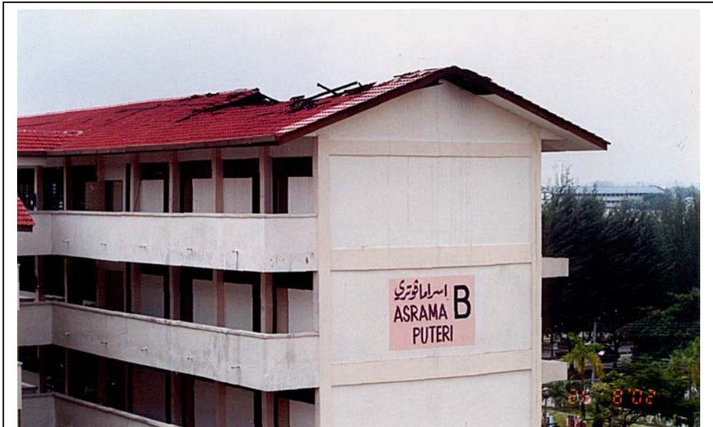
An external view of the lightning damaged hostel of the religious school in Subang Jaya. If the lightning had struck on an occupied dormitory room a few hours later, the possibility of injuries (and even deaths) among the students could not be avoided.
