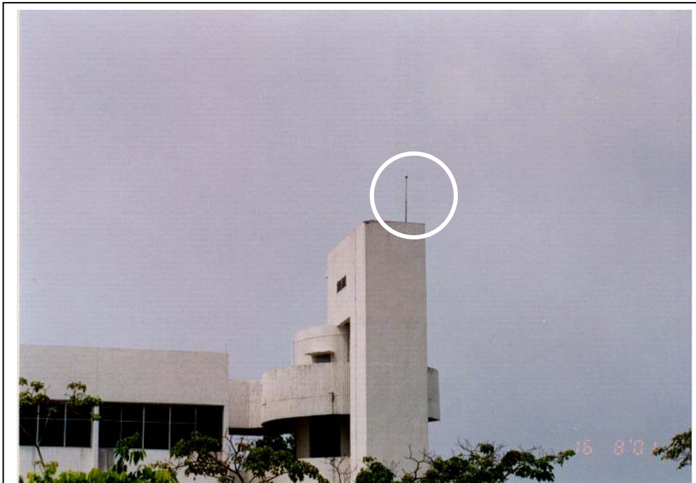
The SIRIM Block #8 with the ESE air terminal (circled) that was installed between January and August 2001. SIRIM still continued to install the ESE air terminals even though the ESE technology had just been dropped from the new Malaysian standard.
