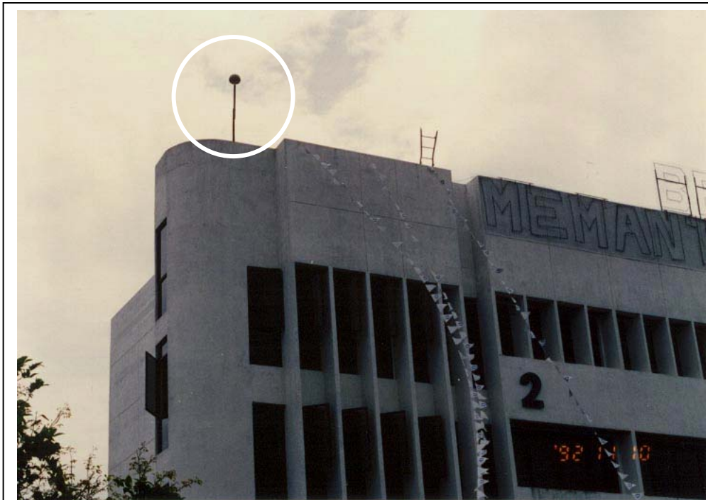
An ESE air terminal (circled) installed on Building #2 of the SIRIM complex in 1992. Another type of ESE air terminal had also been installed on Building #3.
