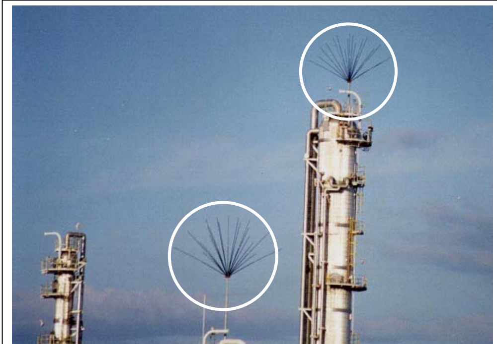
SLE air terminals (circled) installed on petrochemical processing plants in Trengganu. Their claimed ability to reduce the captured lightning current by 99% has been disproved by scientists from the Chinese Academy of Sciences.
