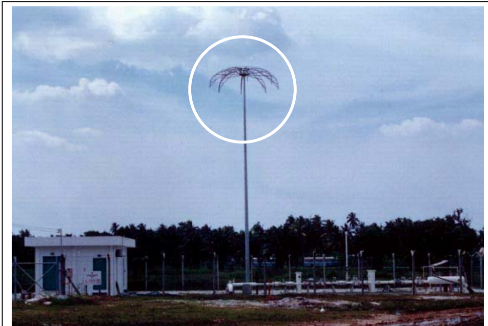
A DAS air terminal (circled) installed at a petroleum gas pumping station in Kapar. Similar installations in the USA have been struck by lightning and have been reported in several scientific papers.
